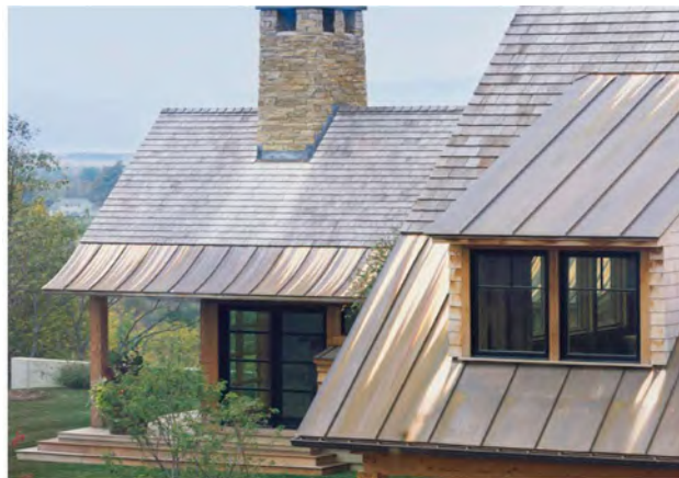
Shake roof and standing seam copper in composition.
