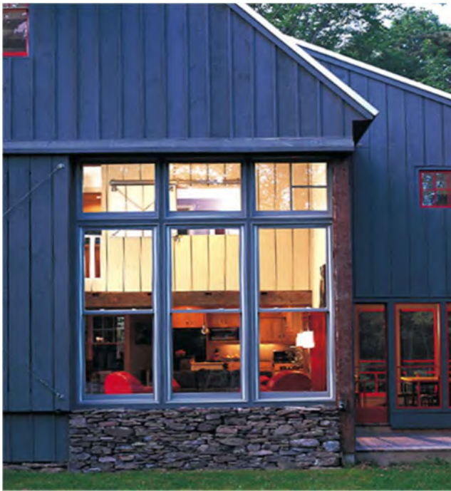
Fiber cement board siding with vertical battens.
