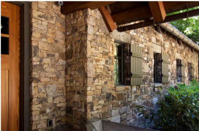
Indigenous dry stack stone exterior.
