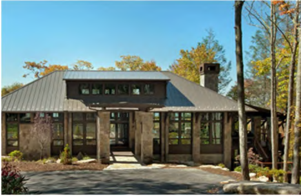
Standing seam metal roof with low sheen.
