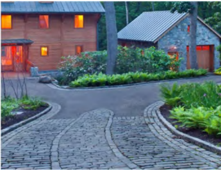
Banding asphalt driveway with stone.
