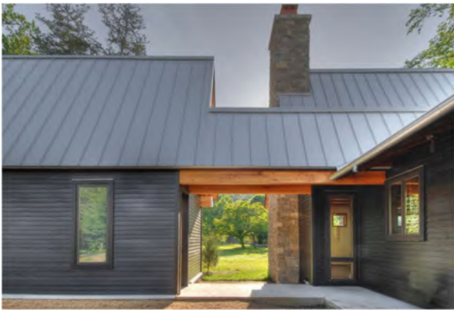
Wood siding oriented horizontally.
