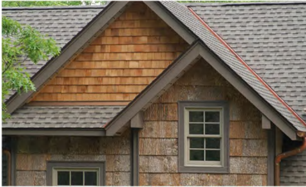
Natural bark siding and natural shingle siding.
